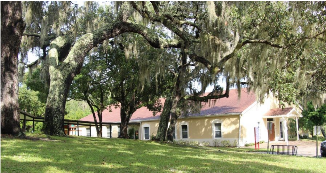
Parish Hall, with covered walkway up to Church building
